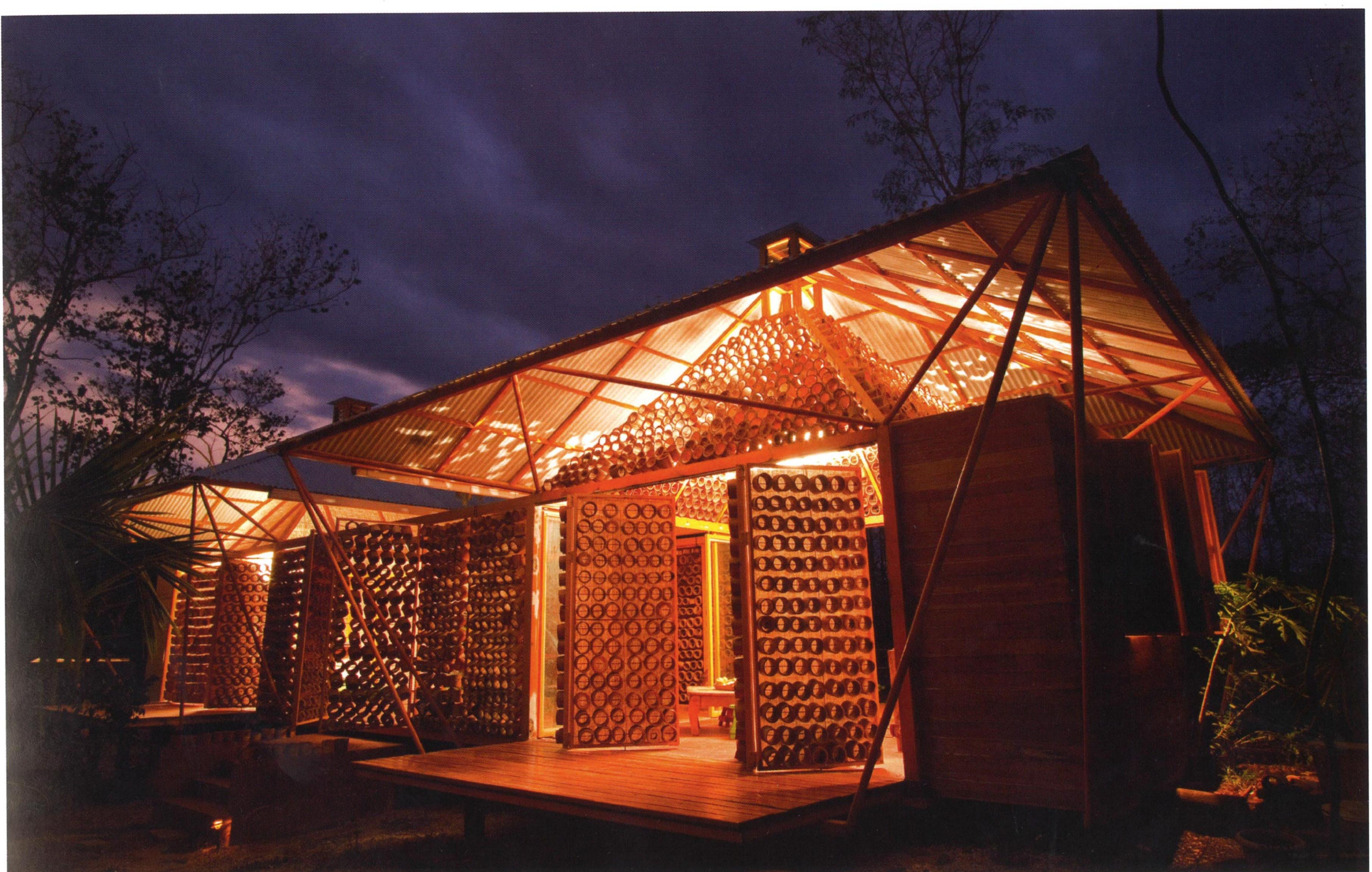
Rainwater is collected, stored and used in the house. The skeleton of the building has two main enclosed spaces and a courtyard in between (opposite). The porous facade facilitates air circulation through the home (top) and allows the home to glow at night (bottom).
